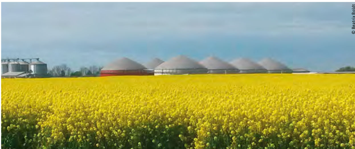
In biogas plants, microbes ferment energy crops and liquid manure to biogas.
