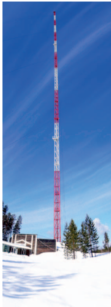
Fig. 5: The Zotino Tall Tower Observatory (ZOTTO) in central Siberia, where long-term measurements of atmospheric composition are conducted at a remote site in the middle of the Asian continent. (Source: Max Planck Institute for Biogeochemistry, Jena)
