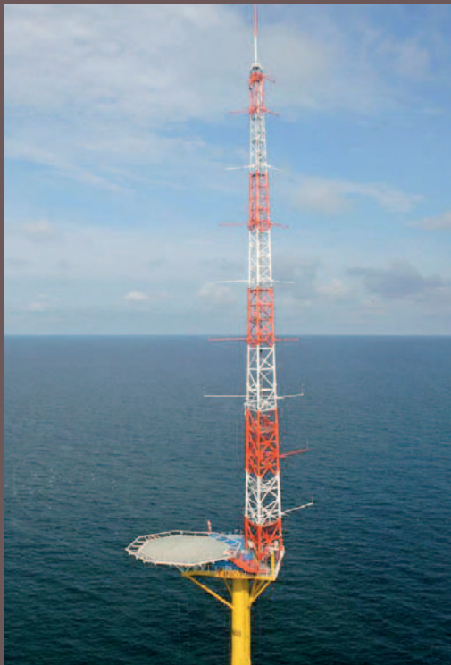
Fig. 15: FINO3 – research platform in the North Sea ( WWW.FINO3.DE ).
