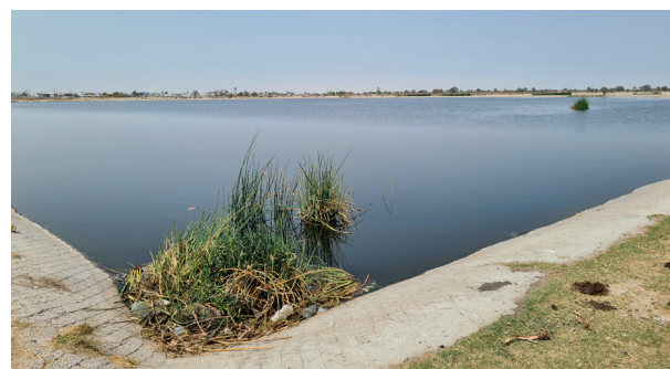
Sewage pond in Oshakati: A typical method used in many communities in Namibia. The ponds are often too small, meaning they frequently overflow during the rainy season.
