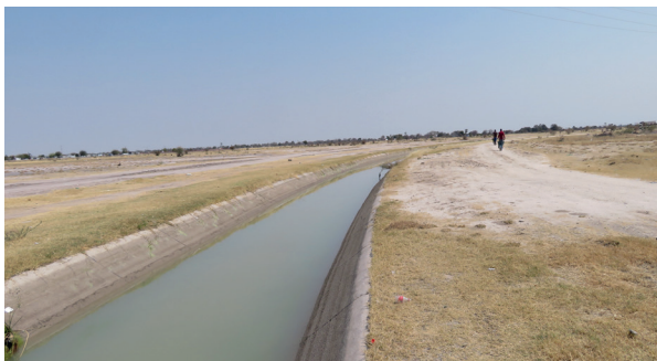
Diversion channel from the Cunene to the Cuvelai catchment in northern Namibia
