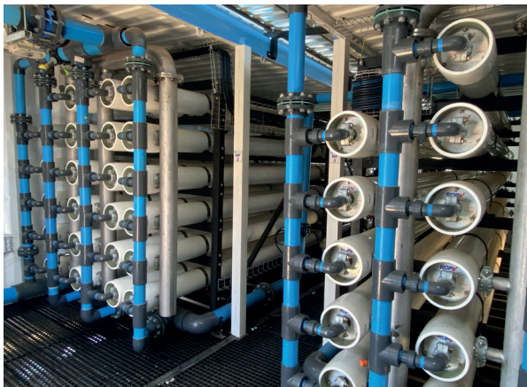
Nanofiltration modules are tested as part of the MAMDIWAS project to investigate the efficiency of membrane technology in mine water desalination.
